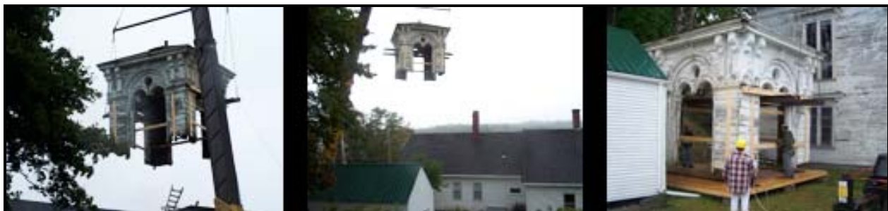
Exterior renovation of historic Liberty Hall included removal and repair of the cupola. Exterior renovations will be completed in 2009. When interior renovations are complete the hall will once again be available for community events and meeting space.
